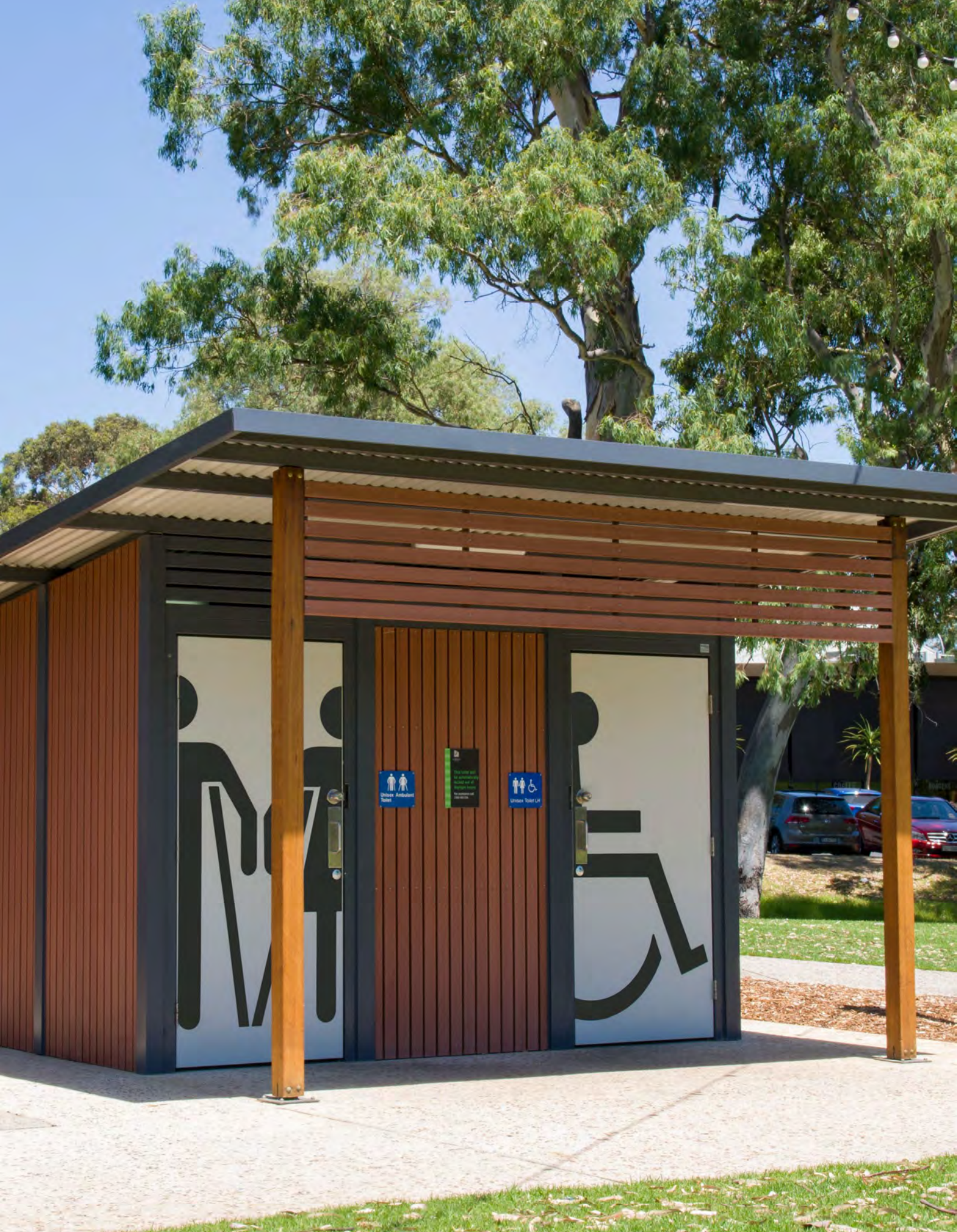
Toilet Block, Civic Park, Modbury
