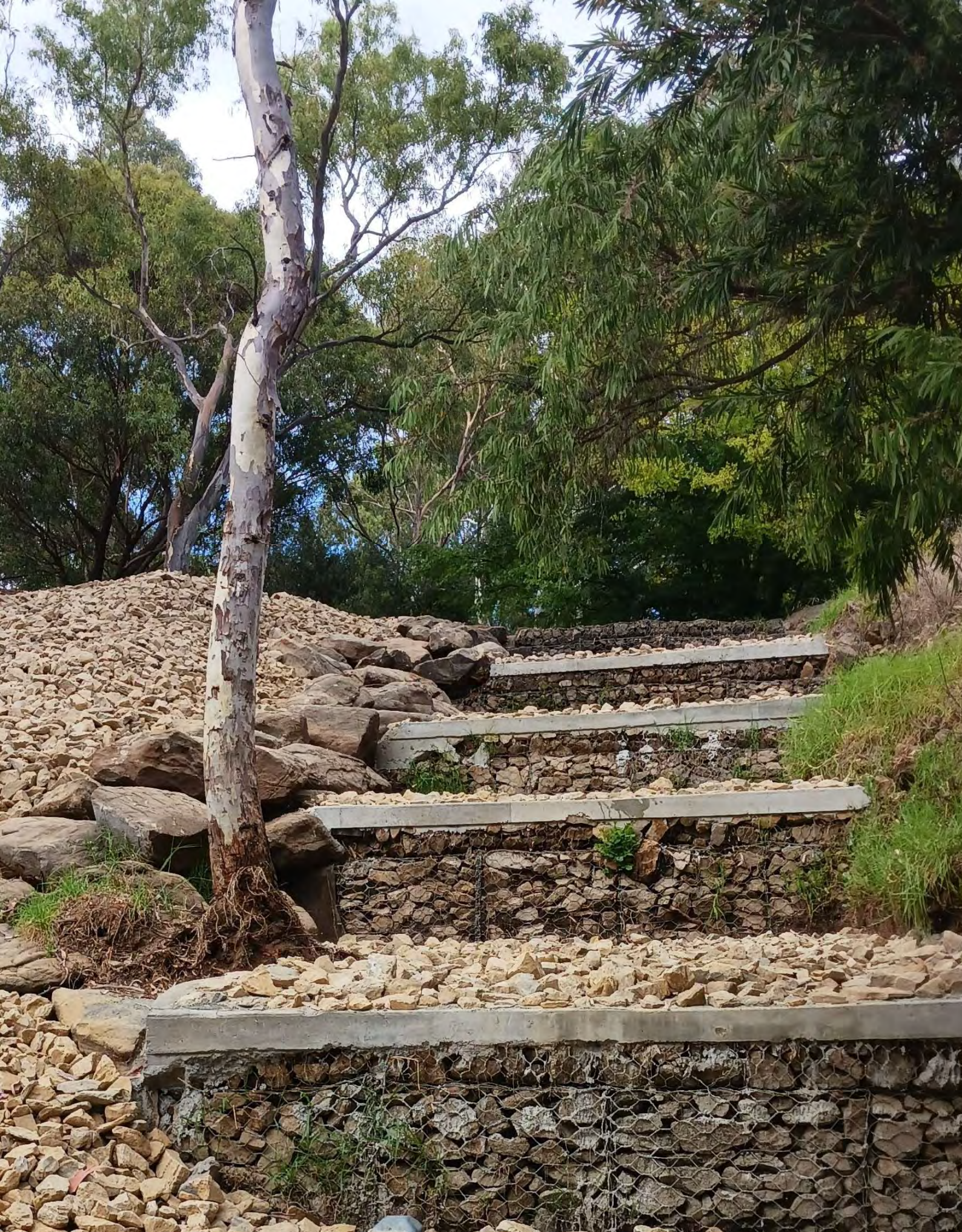
Tiered gabion structure, creek rehabilitation, Cobbler Creek East Reserve, Golden Grove
