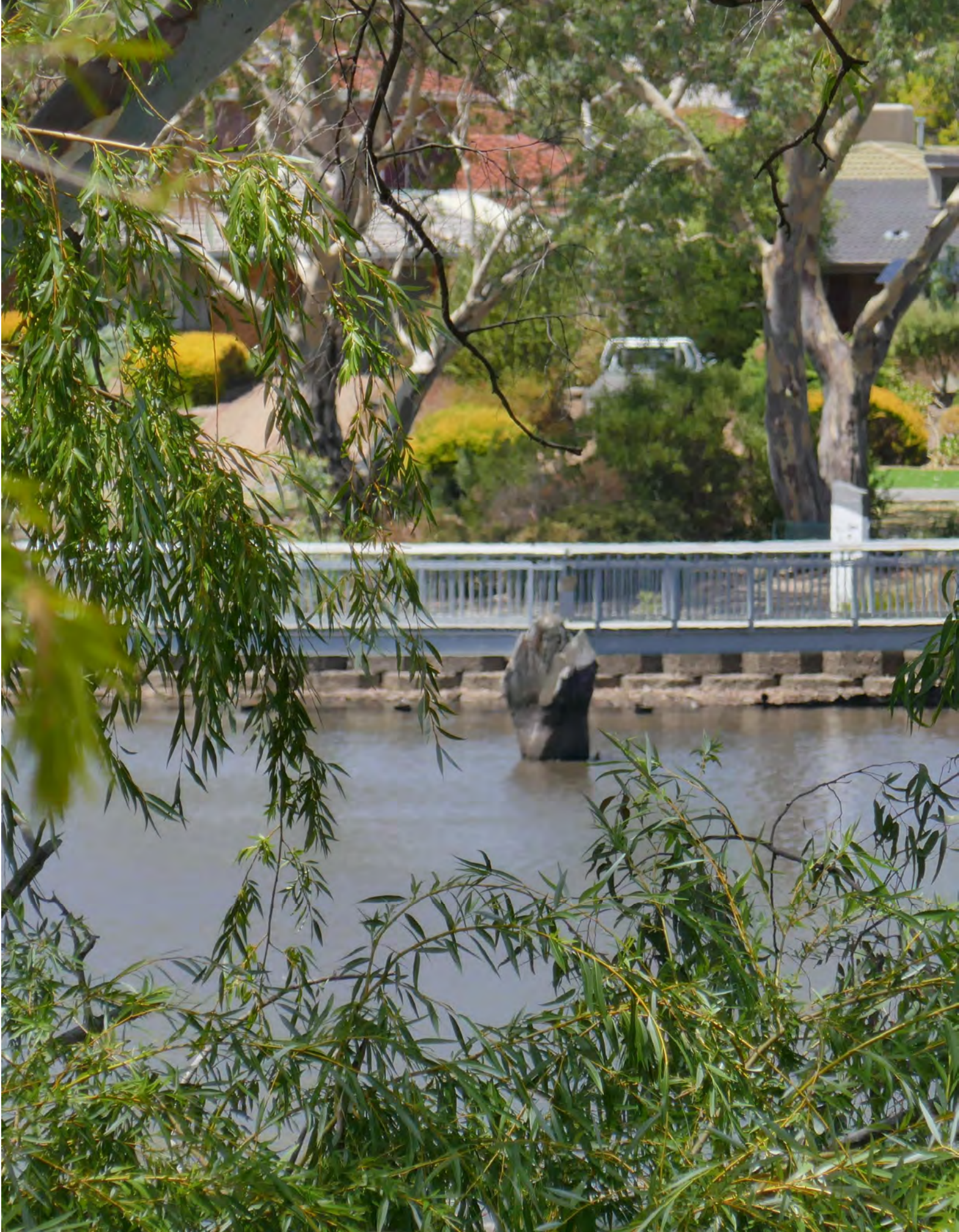
Wynn Vale Dam, Wynn Vale
