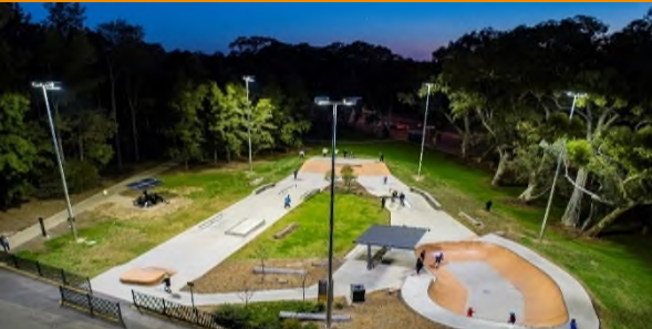
Energy efficient LED public lighting at the Modbury Skate Park, Ridgehaven (Credit: Sports Lighting SA.)
