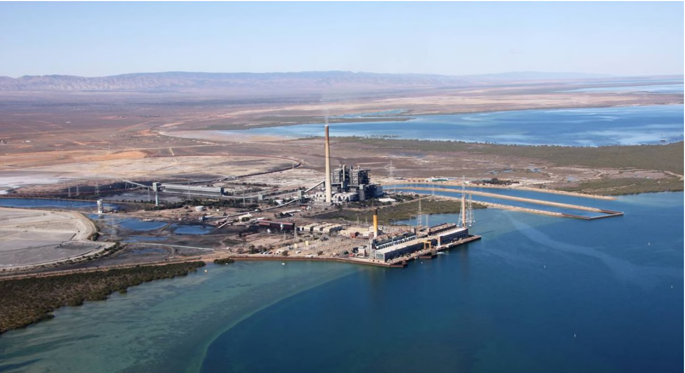
The transition away from thermal coal for energy production has had a marked impact on greenhouse gas emissions in South Australia. The Playford B Power Station and Northern Power Station (pictured), both near Port Augusta, were the last coal-fired power stations operating in South Australia, ceasing operation in 2016. (Credit: Port Augusta Operations).
