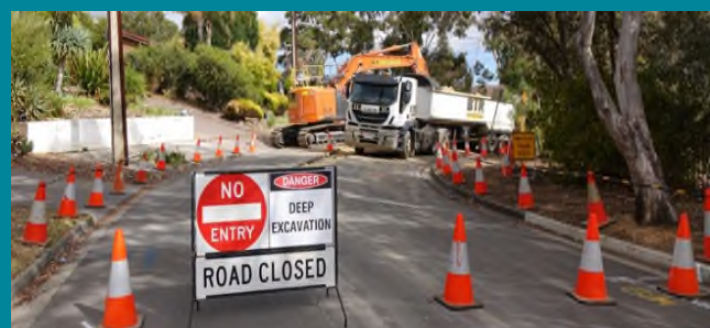
Construction of a sewer main in Banksia Park. (Credit: SA Water.)
