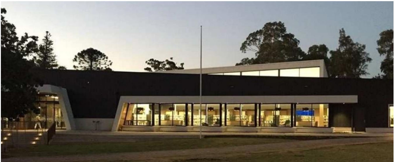
Example project: Mitcham Library and Brownhill Creek redevelopment, City of Mitcham
