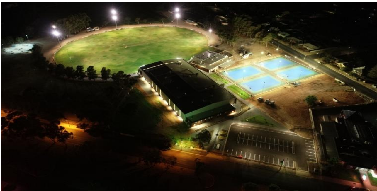
Example project: Loxton Sporting Centre Precinct, District Council of Loxton Waikerie
