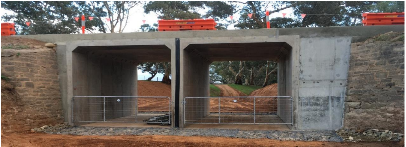
Example project: Mt Allen Road Bridge Replacement, Light Regional Council
